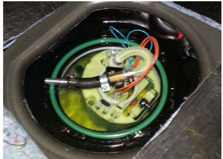
Pump Assembly Into Tank
