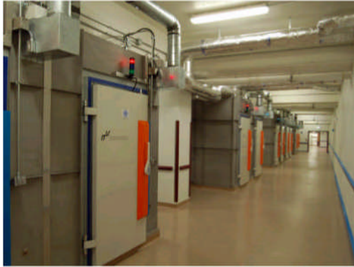
Figure 1. Half of the 21 chamber installation.
