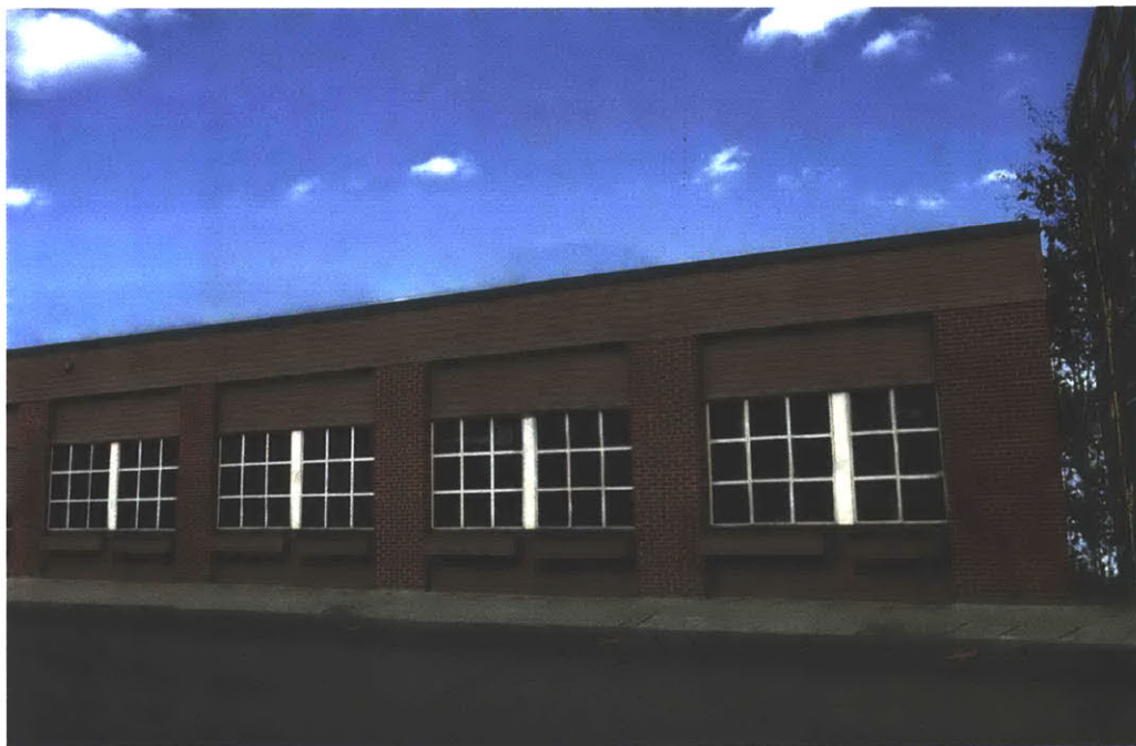
Figure 4-16: The cars and street details have been removed. This example took less than 10 minutes.
