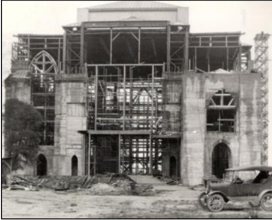
St. Mark's Cathedral under construction, 1930
