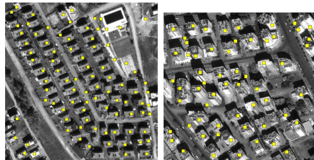
Fig. 11. Building detection results by decision fusion in the Adana 18 and Adana 23 satellite test images.
