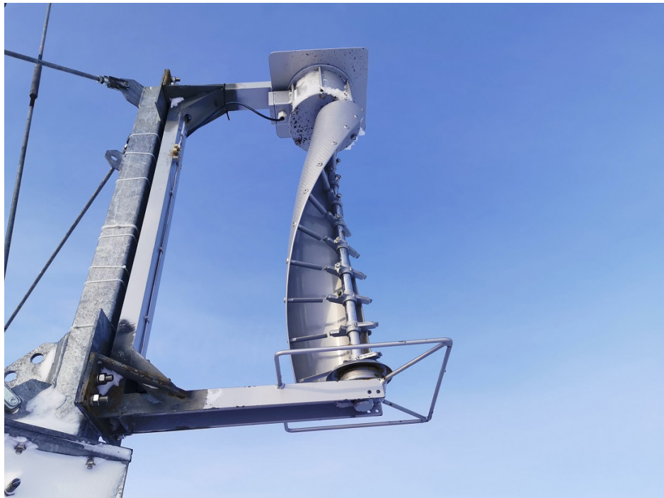
Fig. 4.6.2: SPOT wind turbine damaged during a heavy storm in August 2021
