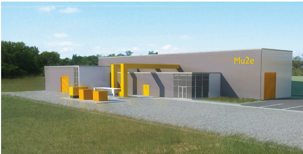
Figure 1.2. Depiction of the above-grade portion of the Mu2e facility.
