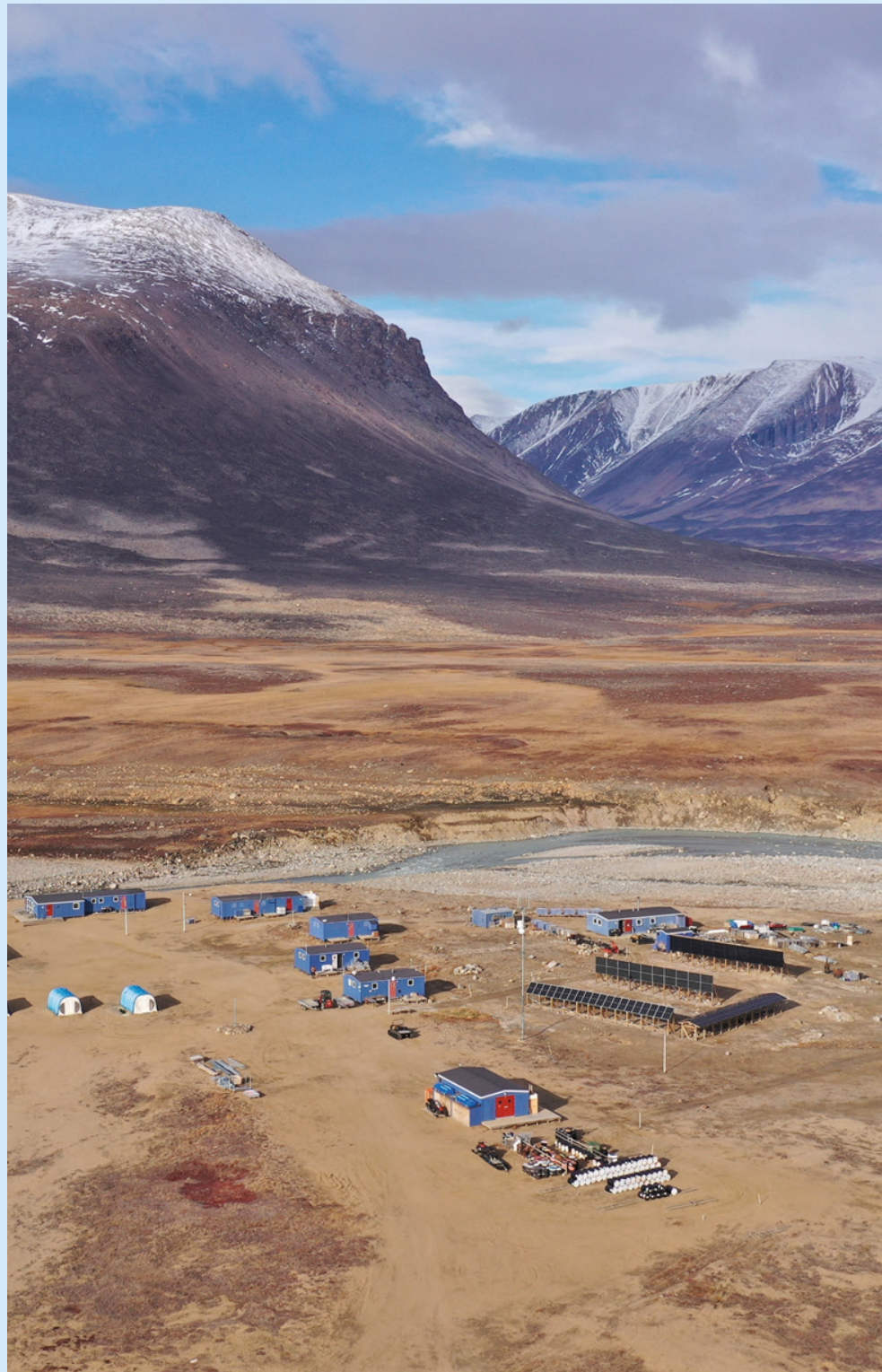
Solar panels installed as part of a green transition at Zackenberg Research Station, Greenland. Photo: Torben R. Christensen.
