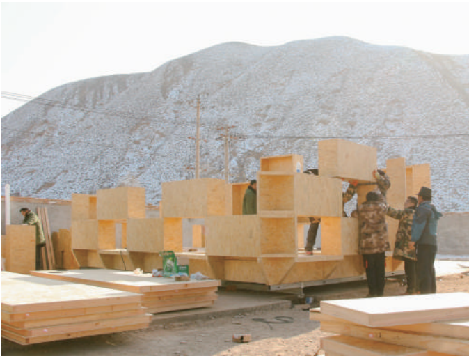
Easy On-Site Assembling of Checkered Playhouse 格子屋現場組裝過程簡易
