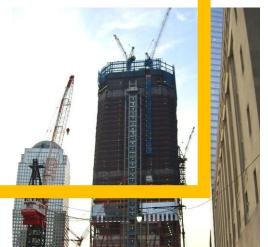
The geometrical shape of the tower reduces exposure to wind loads, as well as the amount of structural steel needed
