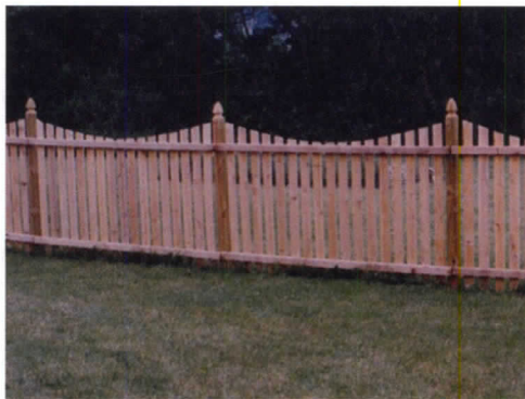
Red Cedar, scalloped spaced picket, 2" space, 4" boards, French Gothic posts
