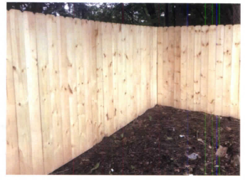
Pressure-treated, Dog-eared solid board, 6" boards, 2" x 4" backing rails
