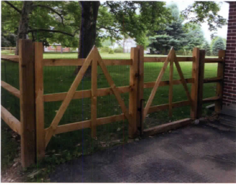
Pressure-treated Split rail, 4-ft tall, 3-rail, double gate, green vinyl wire
