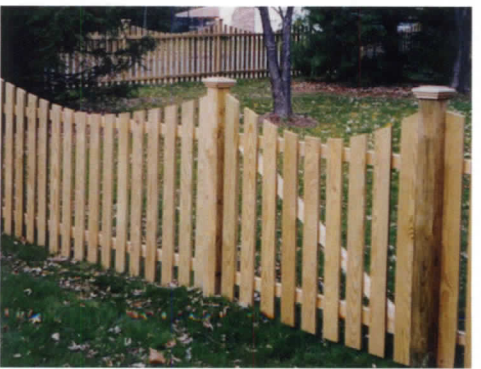
Pressure-treated, scalloped 2" spaced picket with cedar post caps
