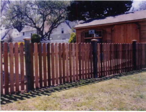
Red Cedar, spaced picket, 1-1/2" spaced dog-eared with cedar post caps
