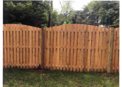
Red cedar, domed shadowbox (tight), 4" boards, 39 per 8' section, cedar post caps (inside view)
