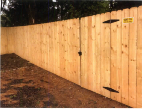
Pressure-treated, dog-eared solid board, 6" boards, 2" x 4" backing rails
