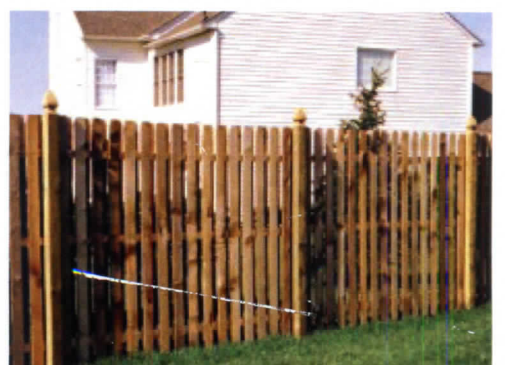
Red Cedar, Dog-eared Boca (regular) shadow box, 4" boards, 33 per 8' section, French Gothic post caps
