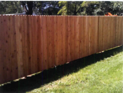
Red Cedar, Dog-eared solid board with 4" boards (outside view)
