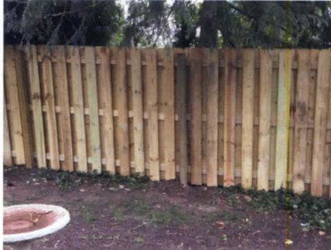
Pressure-treated, Dog-eared, shadow box, 6" lumber, flat top posts
