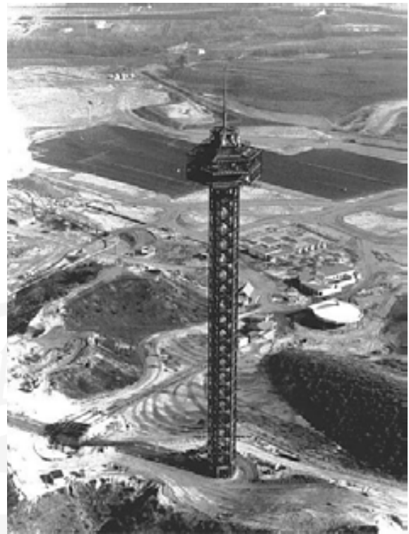
Construction of Magic Mountain-circa 1971
