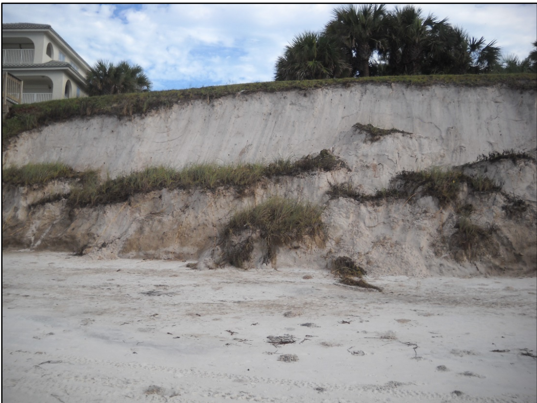
Figure 49. Major dune erosion in Seacrest Beach, R112.5.
