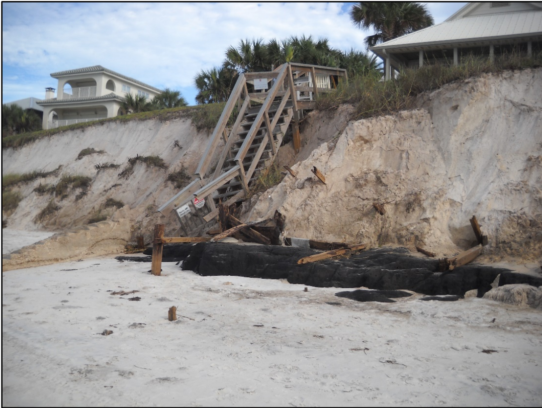
Figure 48. Major dune erosion exposing peat layer in Seacrest Beach, R112.5.
