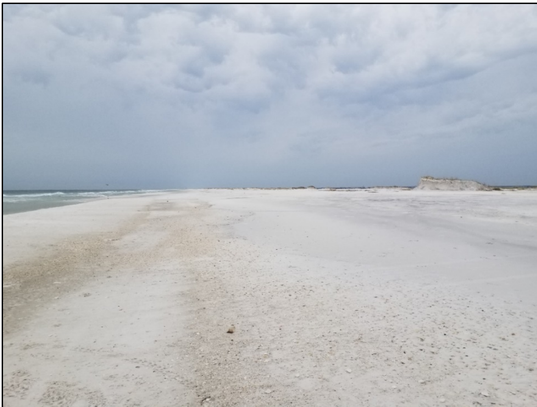
Figure 13. Major dune erosion at Fort Pickens Unit of Gulf Islands National Seashore, R106.
