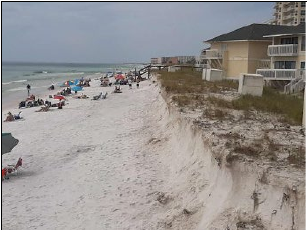
Figure 40. Major dune erosion at Sandpiper Village, Destin, R24.
