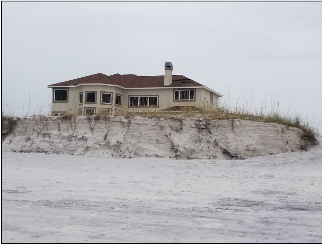
Figure 16. Major dune erosion in Pensacola Beach, R129.
