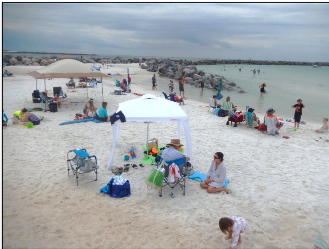
Figure 56. The breach after Tropical Storm Cristobal in June prior to Hurricane Sally.
