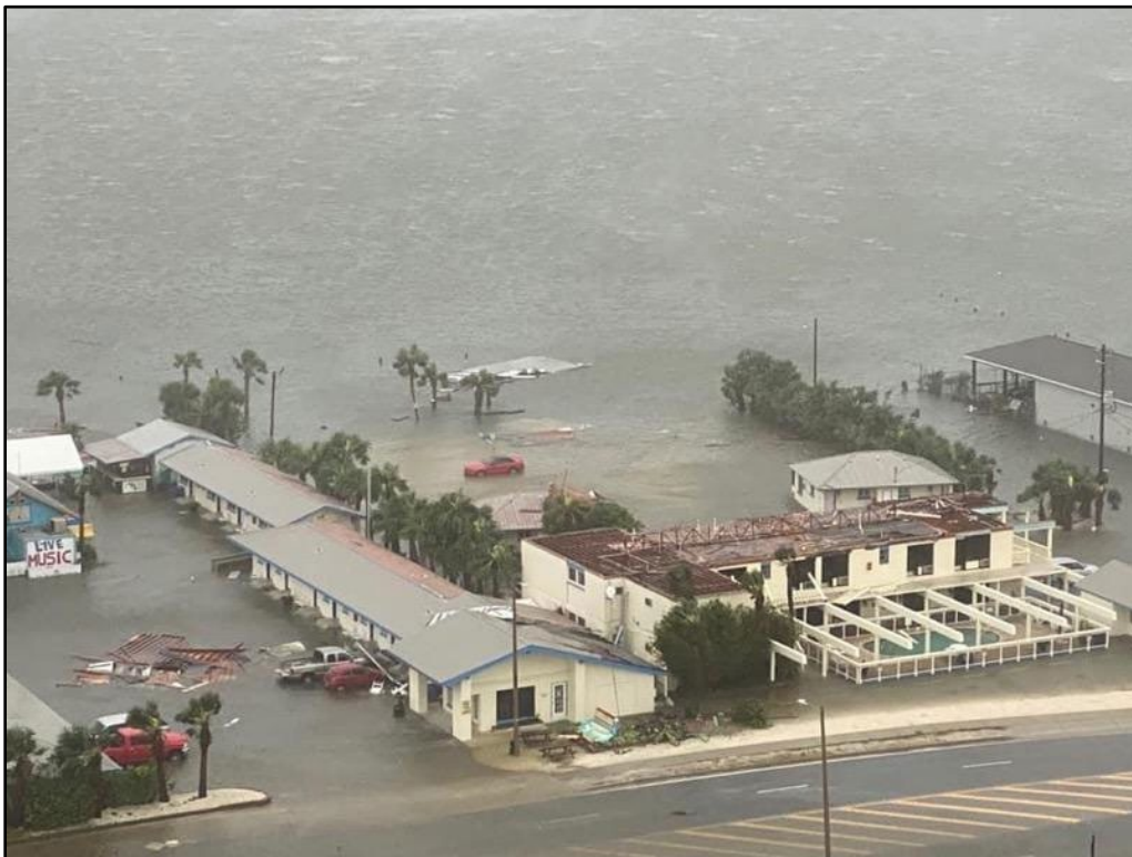
Figure 29. Flooding during the storm at the Pensacola Inn, Pensacola Beach. [Courtesy of Pensacola resident]
