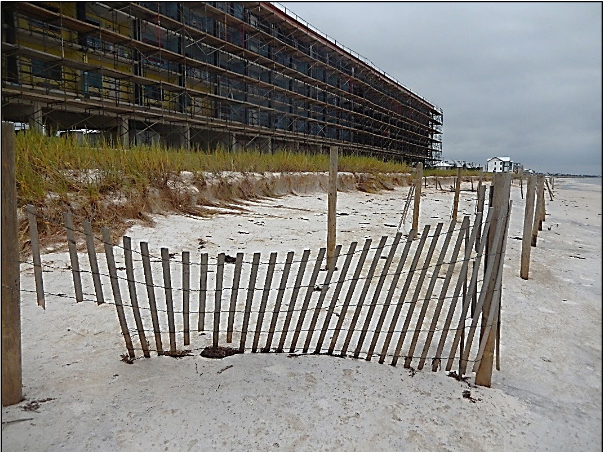
Figure 61. Isolated minor beach and dune erosion (Condition II) in Mexico Beach adjacent the El Governor Hotel (R134.3).
