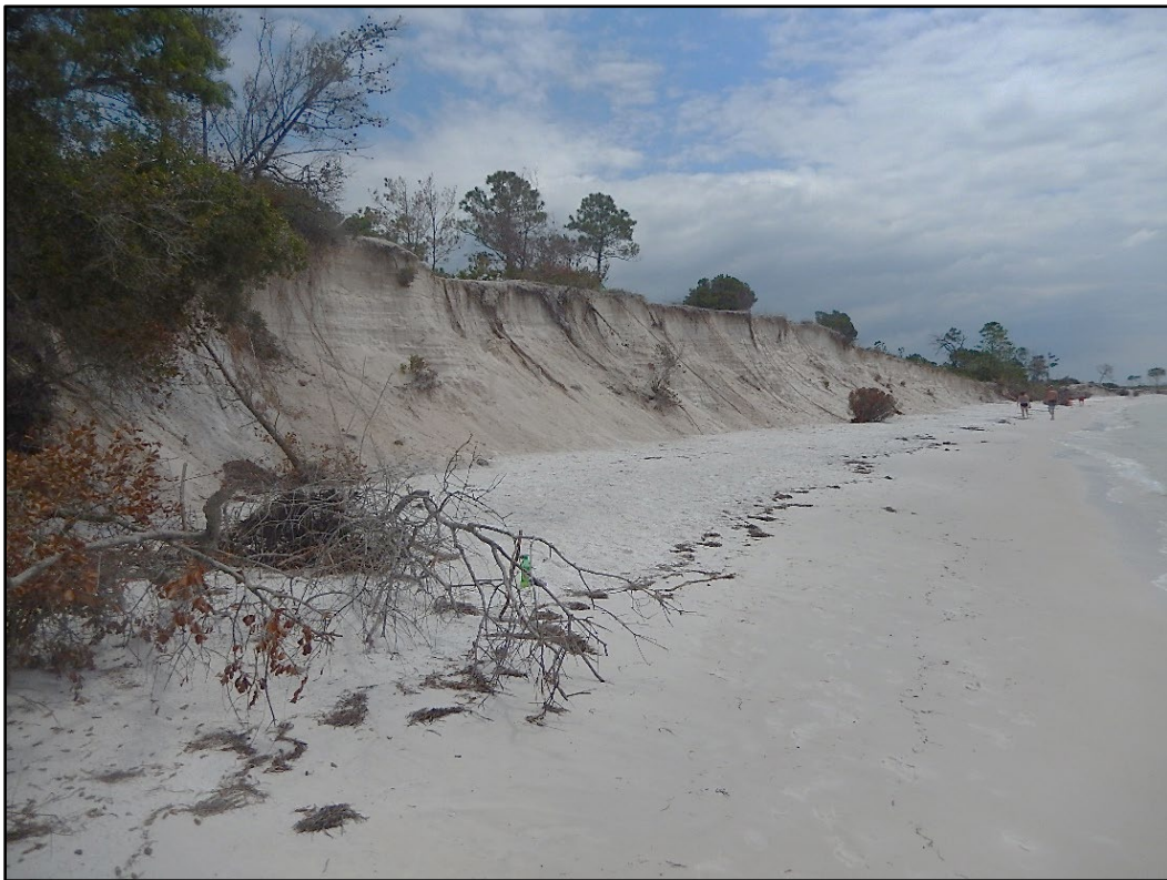
Figure 60. Severe erosion of state park uplands along the west shoreline of St. Andrews Inlet north of the Gator Lake breakwaters and groin.
