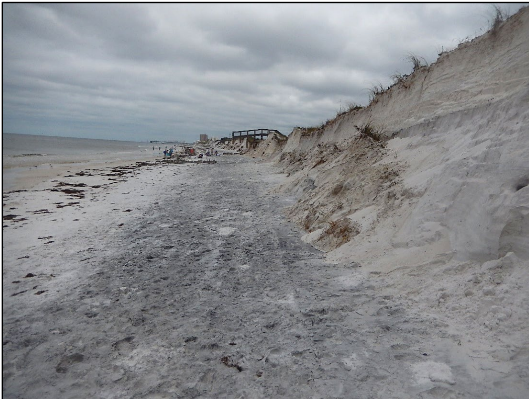
Figure 58. Major dune erosion along St. Andrews State Park (R92-R97) following Hurricane Sally.
