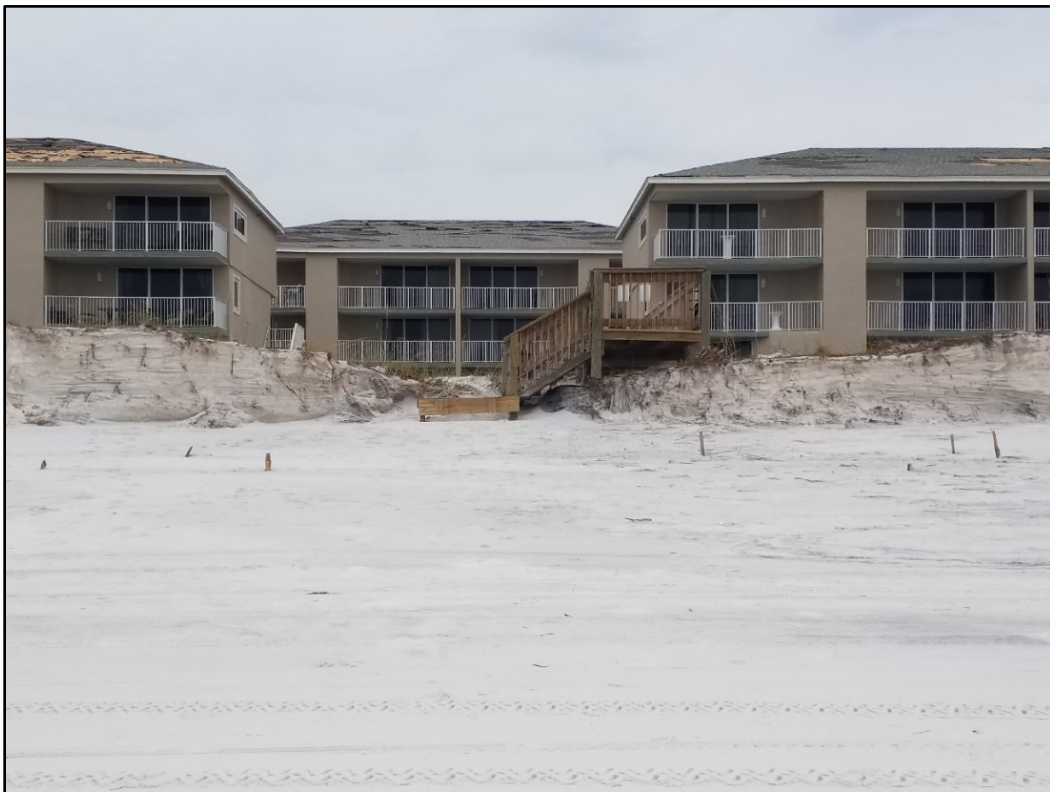
Figure 15. Major dune erosion in Pensacola Beach, R111.
