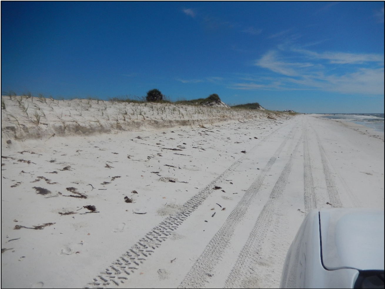
Figure 66. Minor beach and dune erosion at the dune repair section of the Hurricane Michael (2018) inlet breakthrough in the St. Joseph Peninsula State Park (R71-R72).
