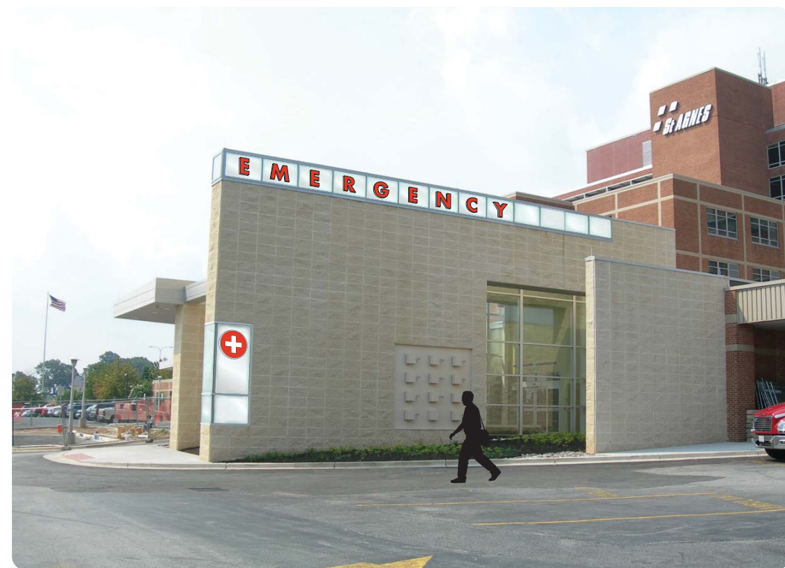
Photo Showing New Emergency Identity Wall Mounted Lettering
