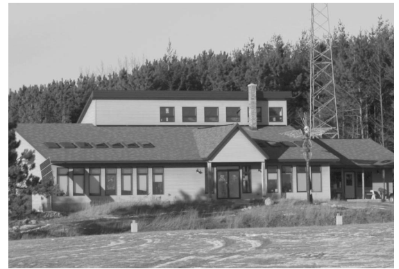
(above) The passive solar features designed into the Midwest Renewable Energy Association's headquarters in Custer, Wisconsin would also work well for a residence. Shown here is the building's southern facade with its many windows. Note the clerestory windows at the top that bring solar energy into the rear of the building. Also, note the small skylights that admit abundant light during the day, but lose a minimum of heat at night. A house with passive solar features like these would not be out of place among conventionally designed houses.
