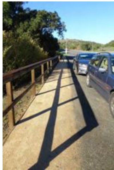
New roadway berm provides safe access to Edgewood Park. © 2017 Kathy Korbholz
