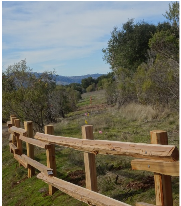
February 2020 – New fencing installed to protect the recovering habitat. Photo © Kathy Korbholz
