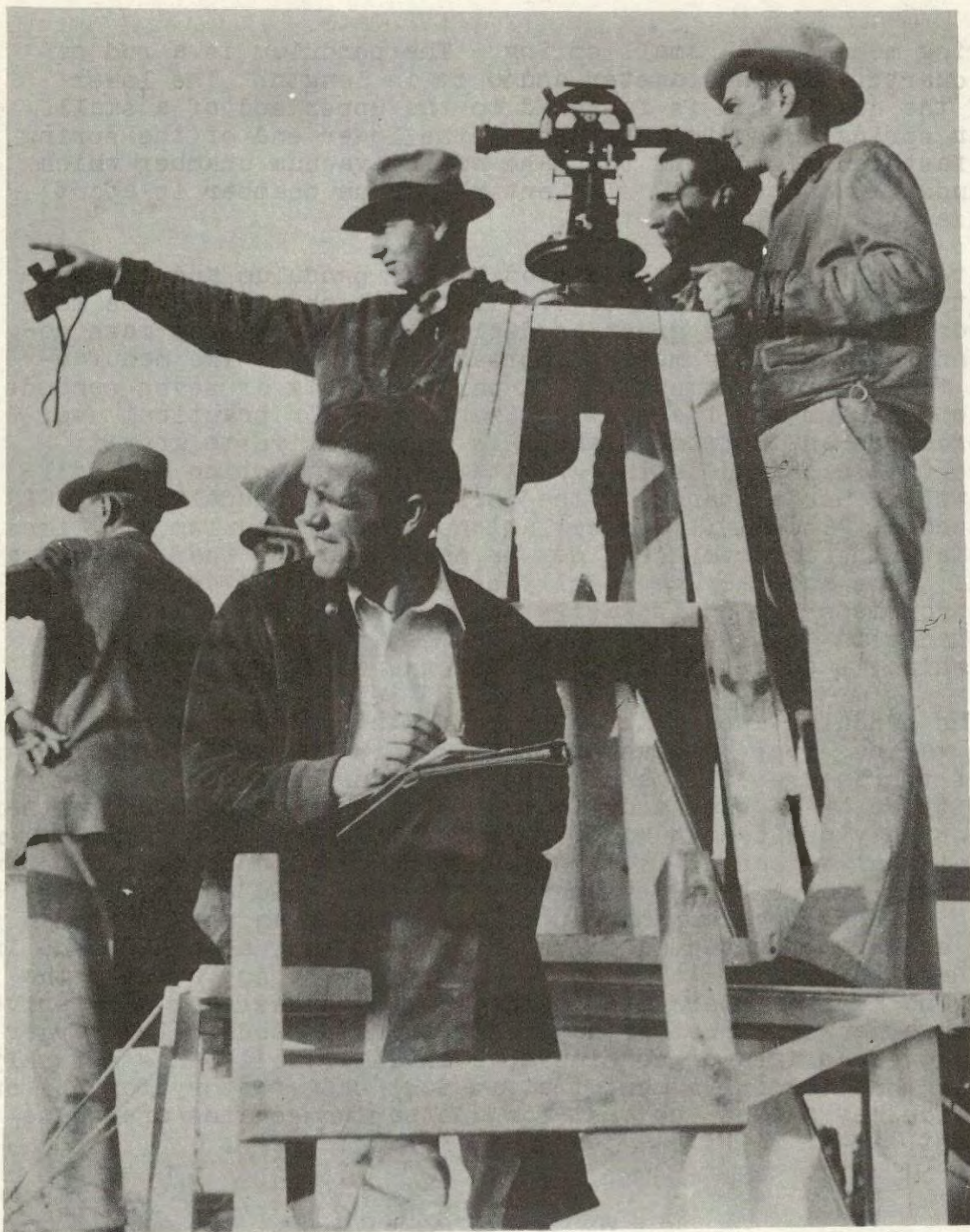
Triangulation party, Coast and Geodetic Survey, occupying top of Washington Monument, 4:00 p.m., Monday, November 19, 1934, access to which was obtained by using the scaffolding constructed to clean this historic structure. The theodolite is placed on a specially constructed stand over the apex as shown.
