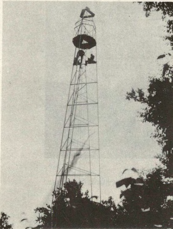
Steel tower completed.
