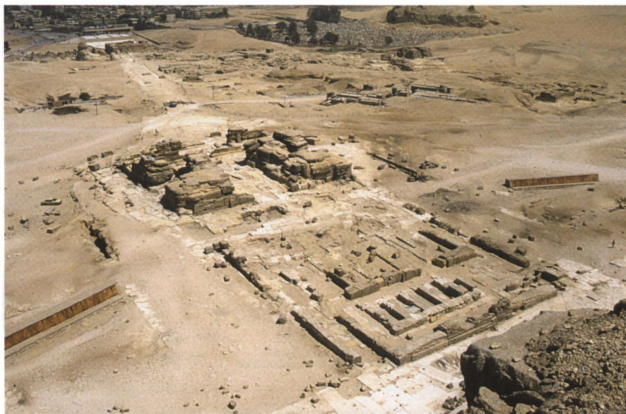
Fig. 98: Mortuary temple of Khafre mainly constructed of local limestone and mud bricks (back). It is cased with fine Tura limestone (foreground) and in inner parts with granite from Aswan.
