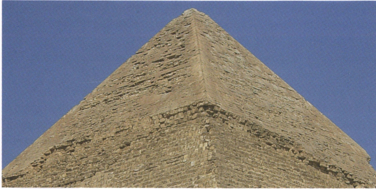
Fig. 96: Khafre pyramid. Remaining casing and backing blocks at the cap.
