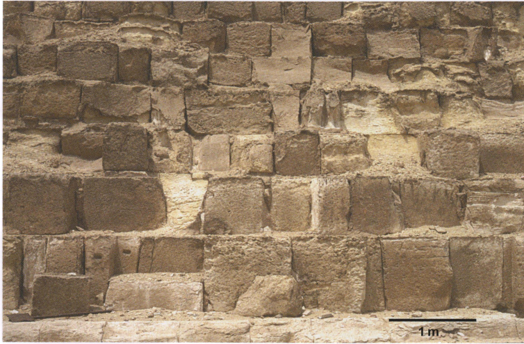
Fig. 86: Block sizes of Khufu pyramid. They differ slightly in width but they are equalized in height.
