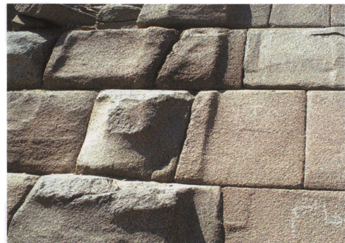
Fig. 105: Detail of Menkaure pyramid. Granite casing blocks at its northern site in various states of smoothing.
