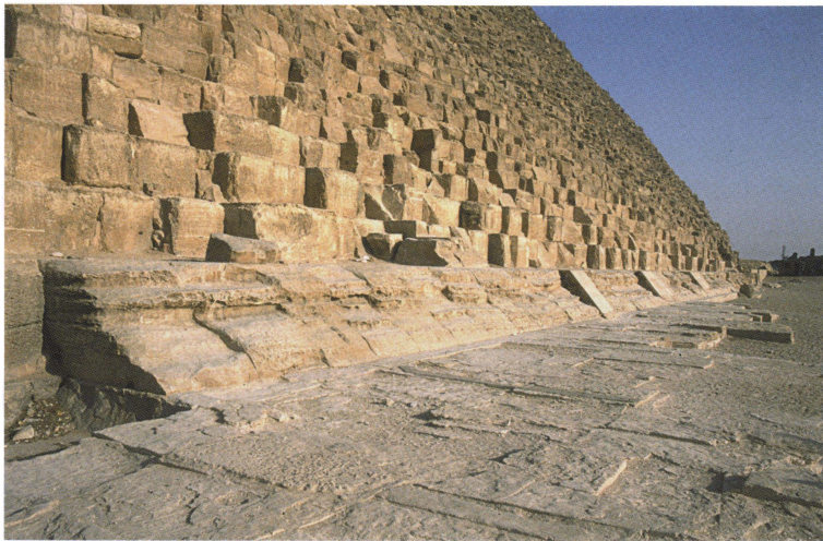
Fig. 87: Casing and backing blocks of Khufu pyramid, western side.
