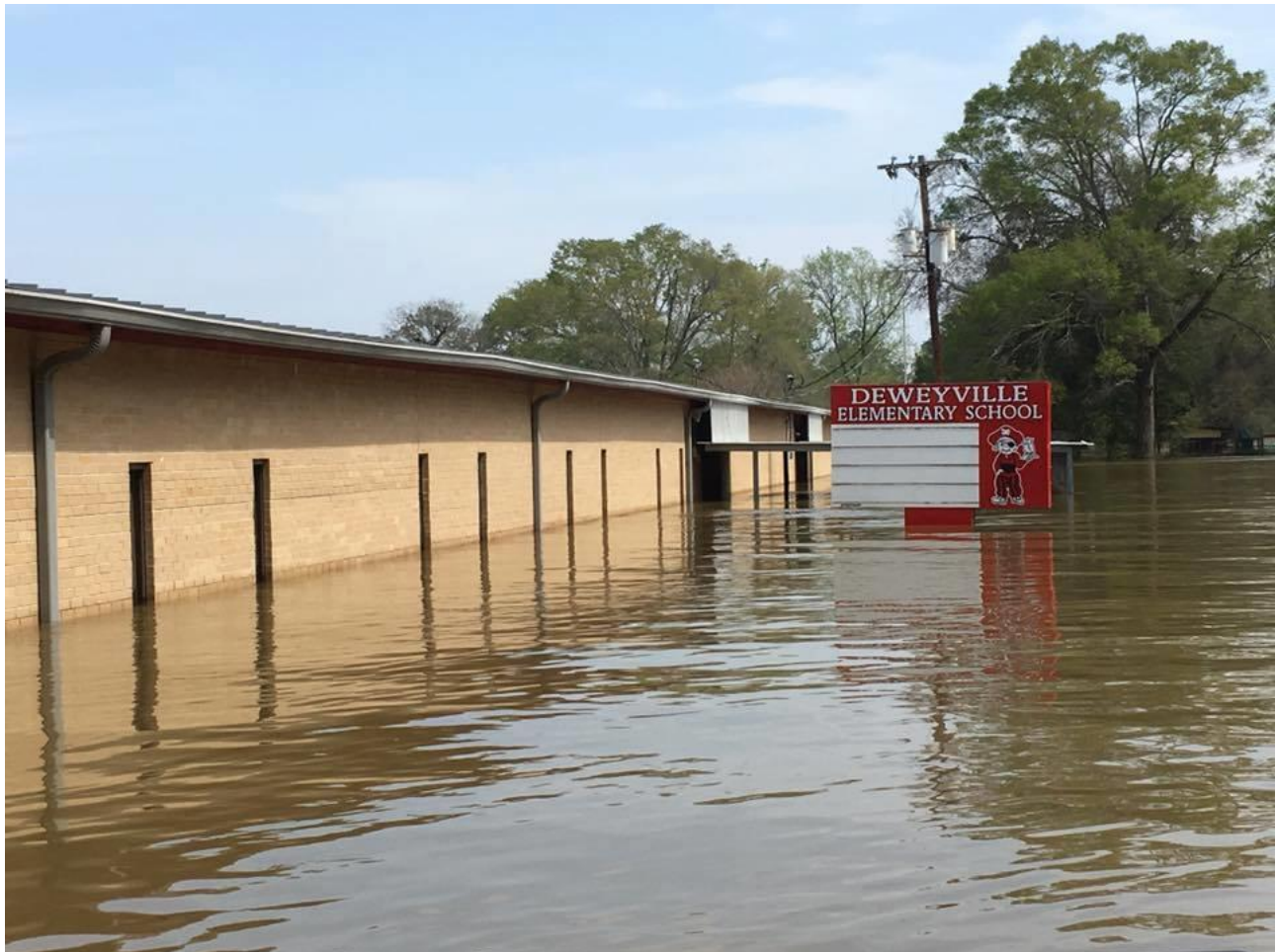
Deweyville Elementary Flooding – photo from Deweyville ISD Facebook page
