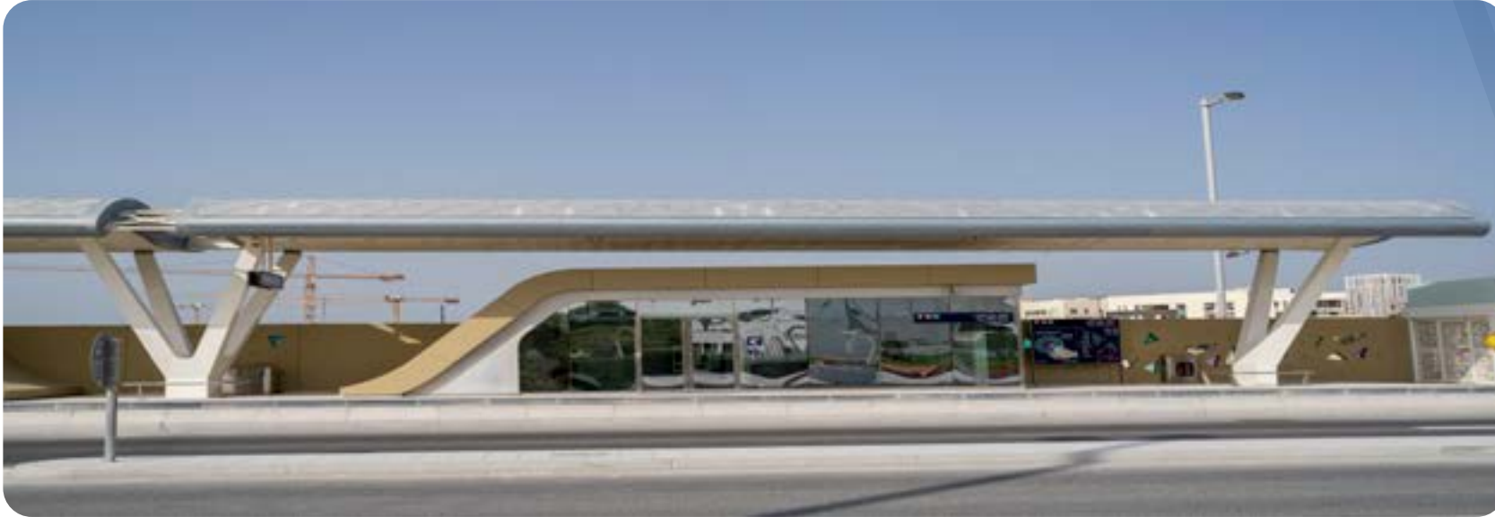
QATAR INTEGRATED RAIL-LRT STATION
