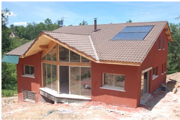
Fig. 1. View of the south facade of the building.
