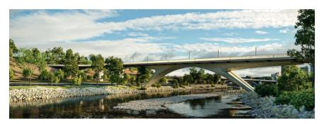
River span with structure above deck (Tied Arch)
