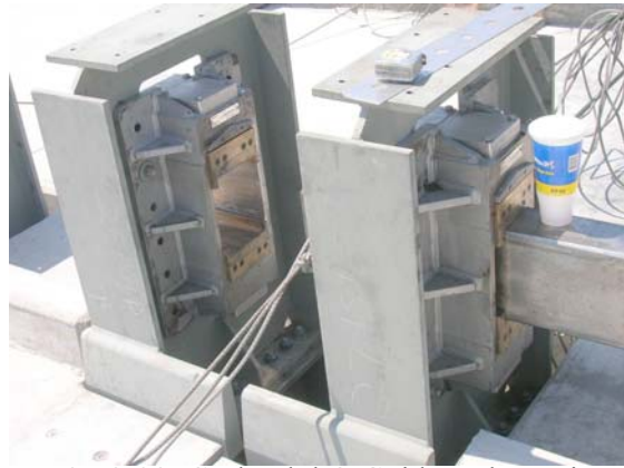
PHOTO 28: Cushionlok® Guide and Receiver
