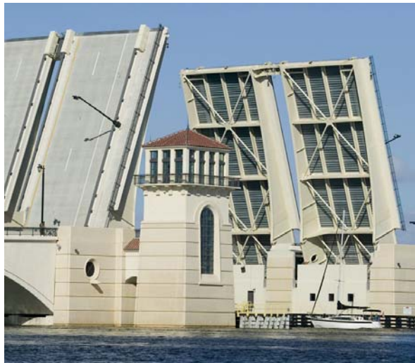
PHOTO 1: Typical Trunnion Bascule Span
