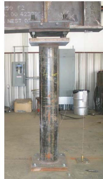
PHOTO 8: Shop Assembly Temporary Support
