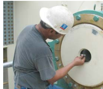
PHOTO 18: Alignment Wire Micrometer Measurement
