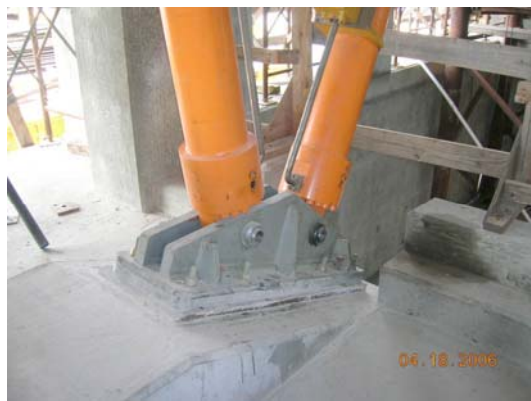
PHOTO 23: Hydraulic Cylinder Lower Clevis
