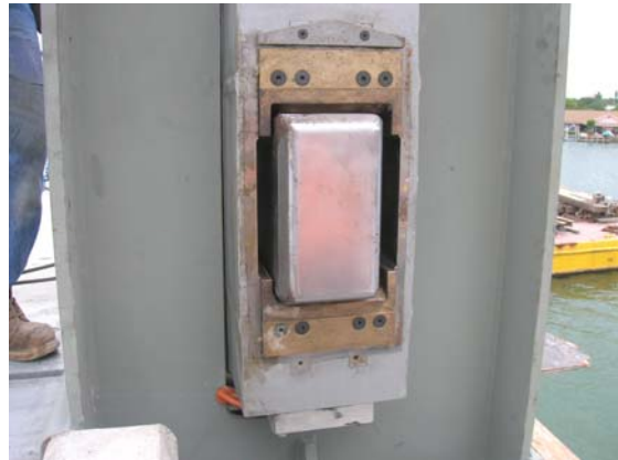
PHOTO 29: Lock Bar End at Receiver
