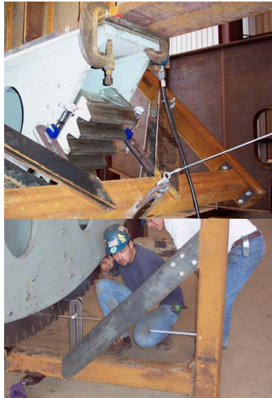
PHOTO 21: Rack Alignment Trammel with Pointers and Dial Indicators
