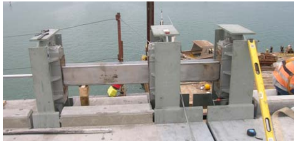
PHOTO 26: Span Lock Bar, Guides and Receiver
