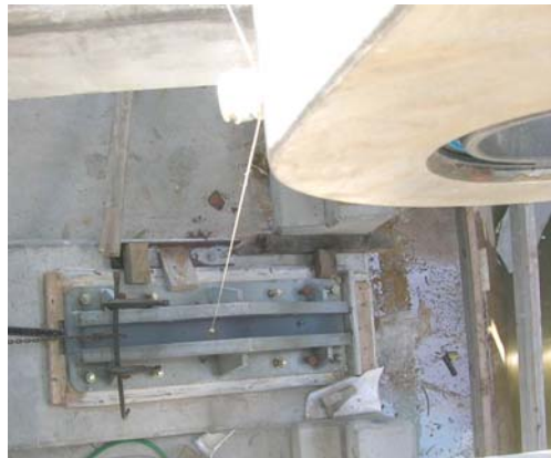
PHOTO 24: Lower Clevis Field Alignment Using Plumb Bob
