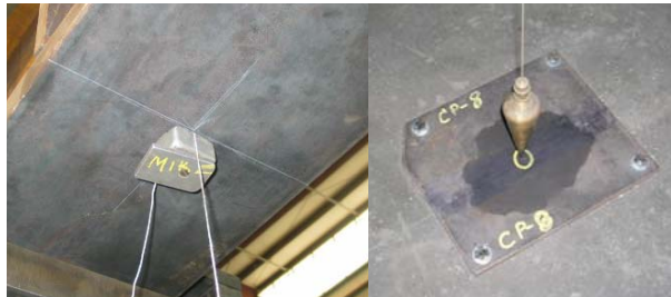
PHOTO 4: Leaf and Floor Control Points
