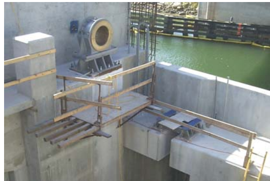
PHOTO 9: Bascule Pier Prior to Erection
