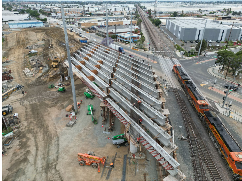
Precast Girders between Abutment 1 and 2
