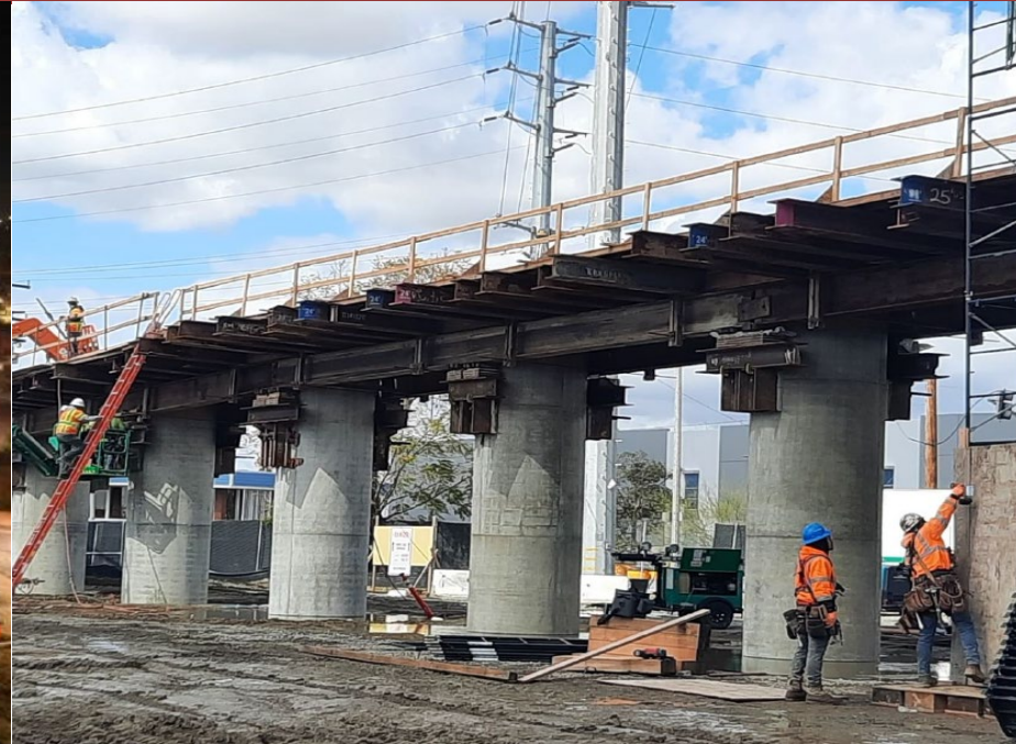
Bent Cap Construction
