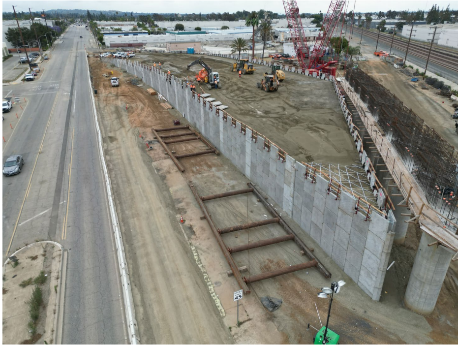
Mechanically Stabilized Earth (MSE) Wall No. 2
