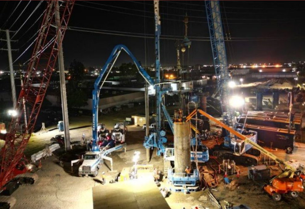
Caisson Installation
