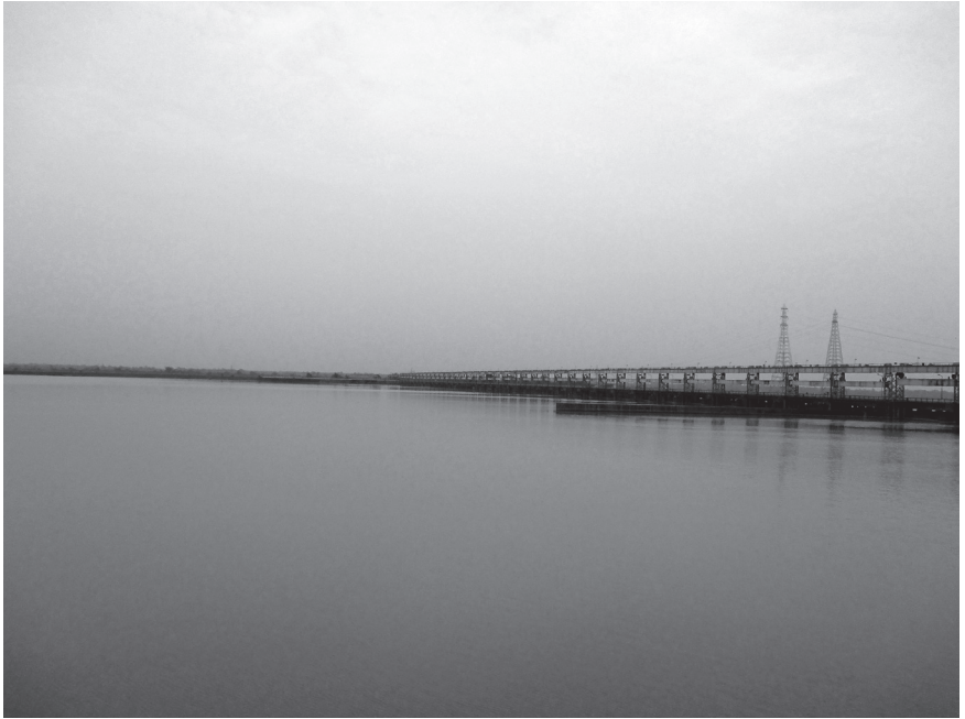
Upstream side of the Gajaldoba Barrage, West Bengal.
