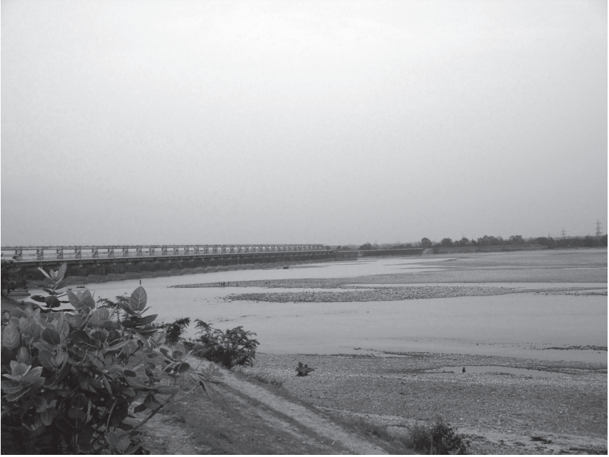
Downstream side of the Gajaldoba Barrage, West Bengal.
