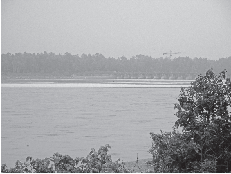
Upstream side of the Dalia Barrage, Bangladesh.
