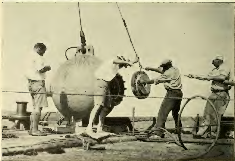
FIG. 82. ( upper ) A thin coating of white lead is placed on the flange of the door to make the junction of steel with steel as perfect as possible. FIG. 83. ( lower ) The door is now lifted and swung gently over the ten great bolts, and the mass of steel clangs home.
