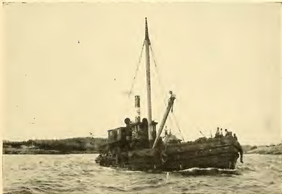
FIG. 65. ( upper ) The giant steel sheaves have been in use for seven years, yet show no signs of wear, and perform their important job smoothly and well. FIG. 66. ( lower ) The Freedom has performed yeoman service in Bermuda for more than twenty years, and she does all that we ask of her. But with our heavy load, in rough seas, she discovers leaks of which she was wholly ignorant, and the first day we have to steam full speed to shore with the water almost at the level of the engines.
