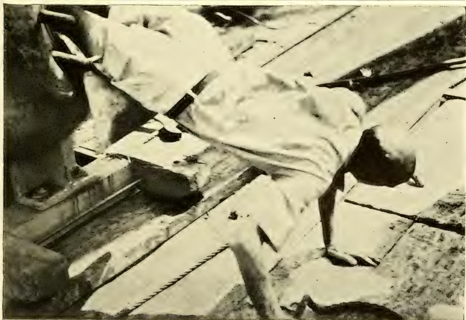
FIG. 96. ( upper ) The wing-bolt is unscrewed, very slowly at the last, when the slightly compressed air hisses out. Through the hole, the more delicate instruments are handed out. FIG. 97. ( lower ) The most painful part of the whole dive for the divers is when they emerge, tired and cramped, with feet asleep, and haul themselves out of the fourteen-inch opening of the door.
