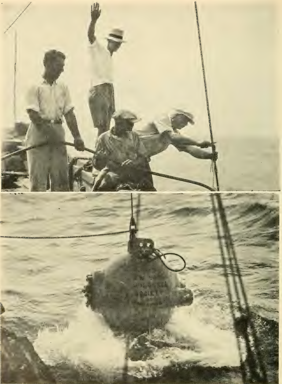
FIG. 94. ( upper ) The greatest depth, 2200 feet, has been reached, and now the bathysphere is on its way up. To save time the rope ties between cable and hose are quickly cut, so there is scarcely a moment's delay at each 100 feet. FIG. 95. ( lower ) Like some great creature of the sea the dark blue sphere breaks the surface, and is held there until there comes a moment of complete steadiness when it is drawn rapidly up, swung inboard and landed.
