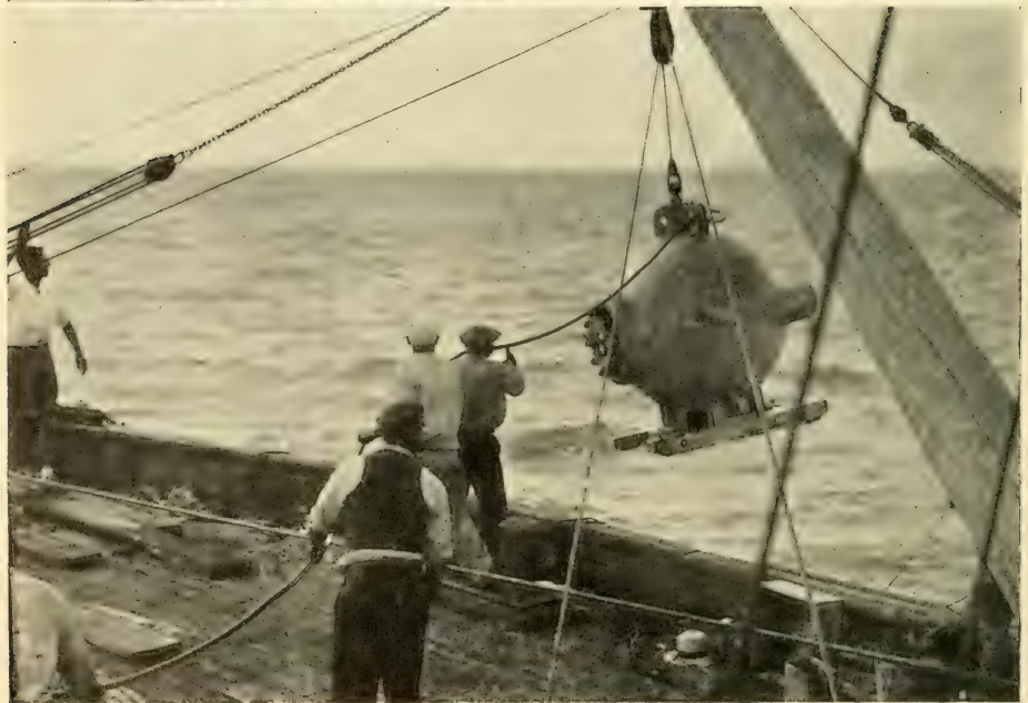
FIG. 86. ( upper ) The door is sealed tight, the signal given, and the two-ton steel ball rises gently, clears the rail and is swung outward. FIG. 87. ( lower ) This is the moment of greatest worry to Tee-Van and Sylvester, who are in charge of the deck machinery. A sudden swell sets the bathysphere swinging like a pendulum; then a second wave counteracts the movement, and at this propitious second, it must be dropped beneath the surface.
