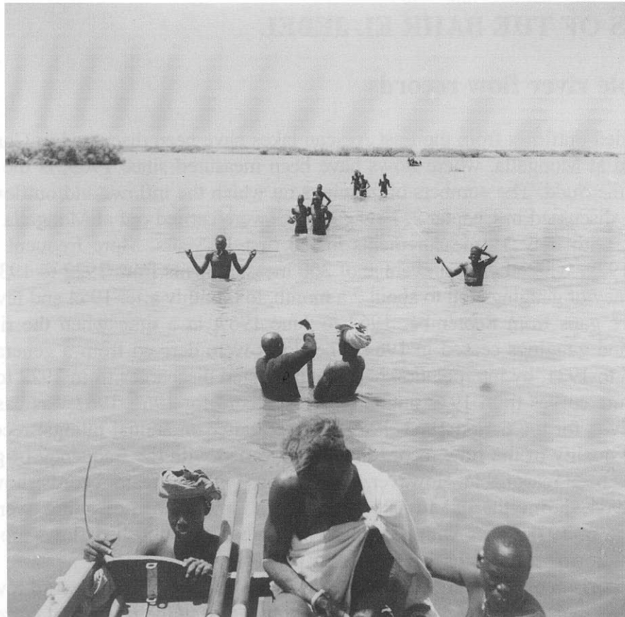
Plate 5 Aliab valley: inserting survey peg on cross-section 15 (cross-section P), February 1951.
