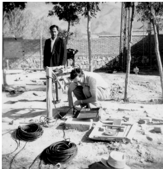
Plate 6.2 Observing water levels during a pumping test northwest of Tehran.
