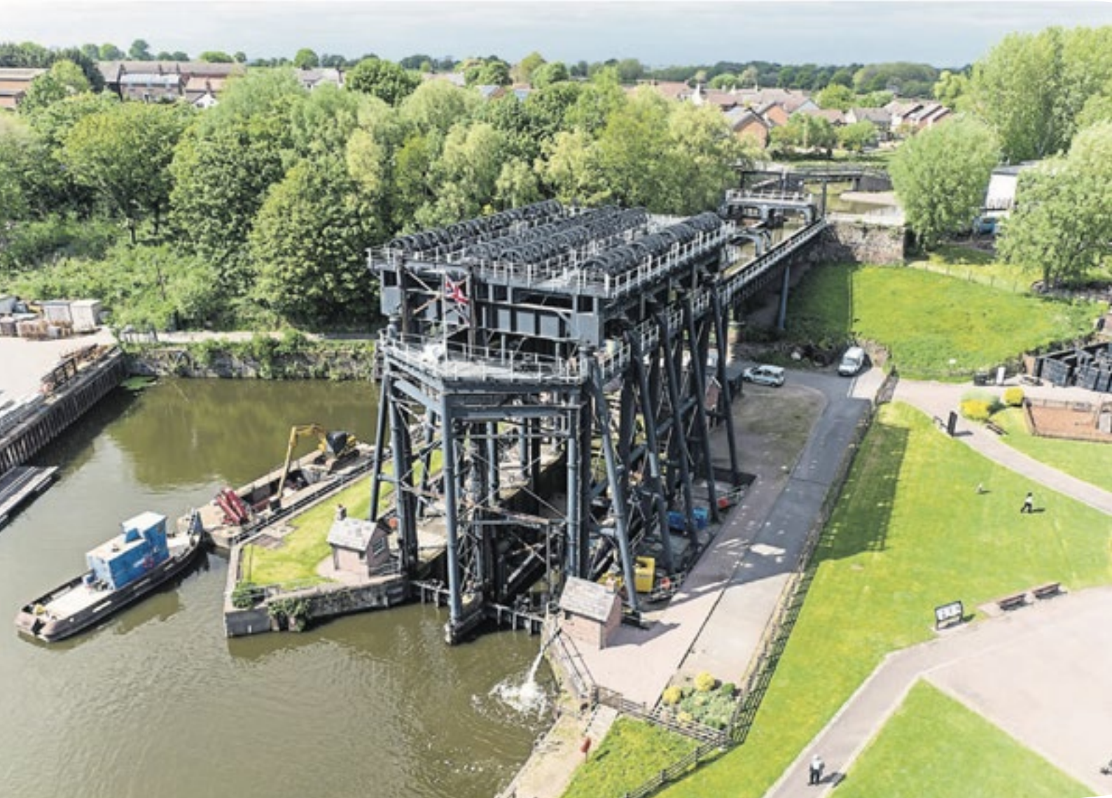
Twenty years after restoration, Anderton Boat Lift needs a major overhaul. Photo credit: Canal & River Trust
