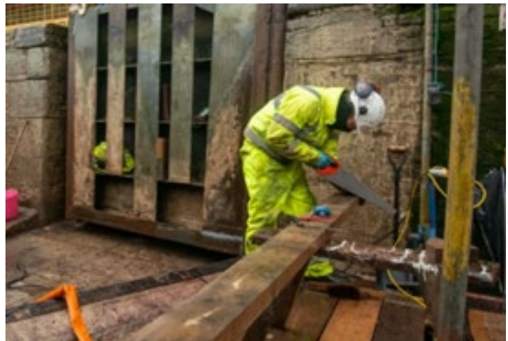
Repair work being undertaken at Caen Hill Flight
