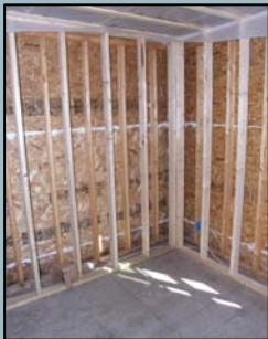
Double walls at an RDI home – before insulation with dense cellulose.
