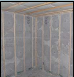
Double walls at an RDI home – after insulation with dense cellulose.
