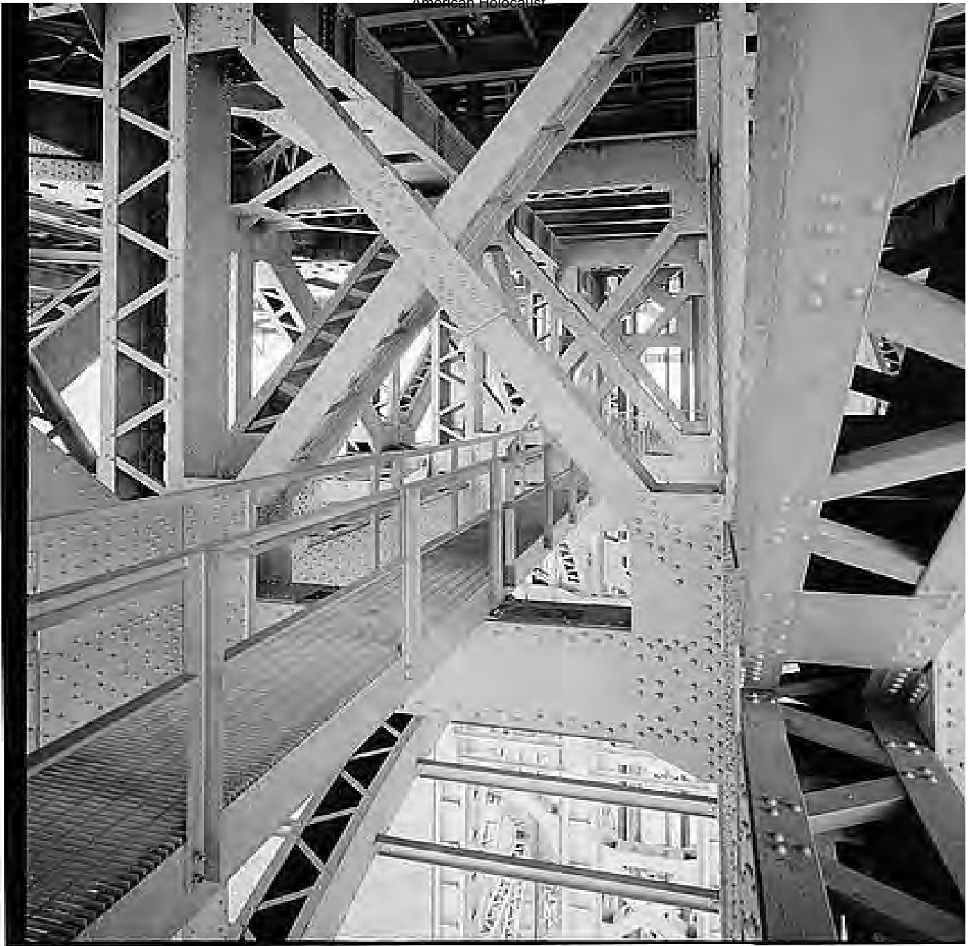
Roadway supports, George Washington Bridge
