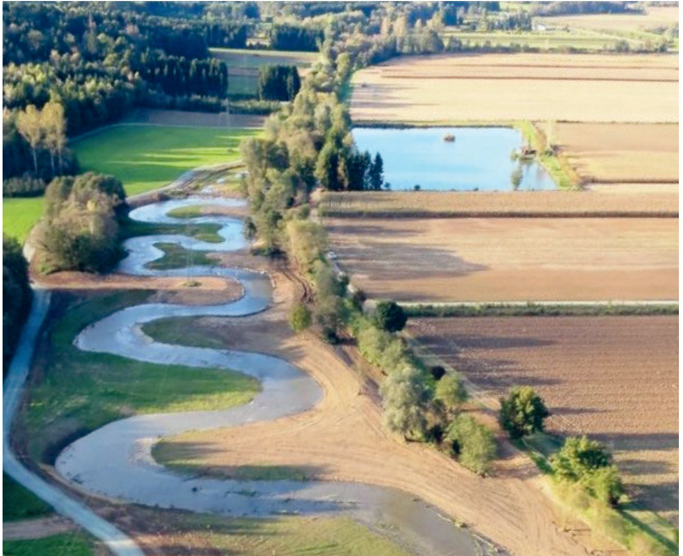
Meanders of the Pinka upon completion of the construction process
