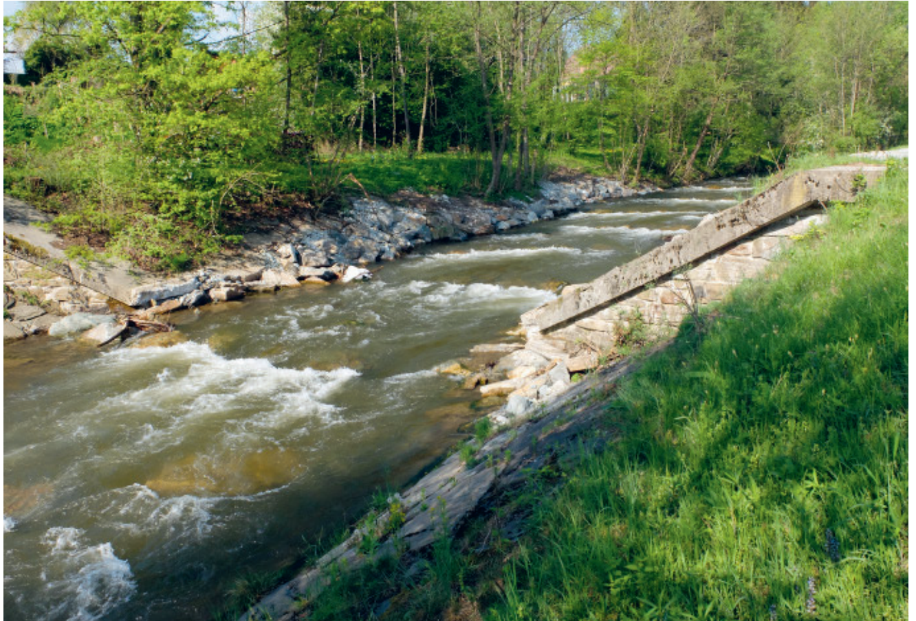
Boulder ramp in the area of the former transverse structure in Gasselsdorf
