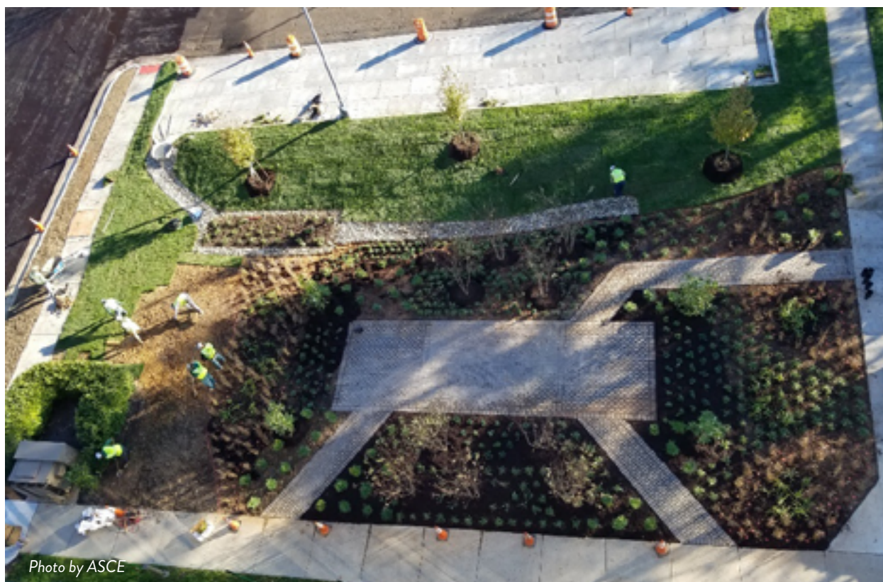
PERMEABLE PAVEMENT AND STORMWATER DETENTION IS BUILT INTO A PARKING LOT IN RESTON, VIRGINIA.
