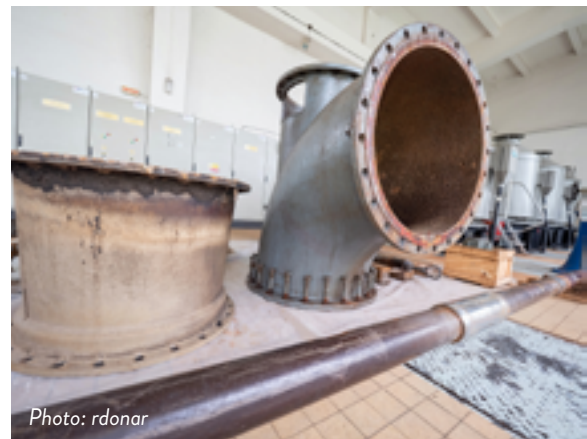
AXIAL HYDRODYNAMIC FLOW PUMP IN WASTEWATER PLANT.
