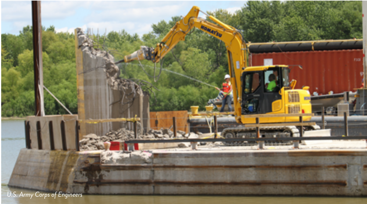
LA GRANGE LOCK AND DAM ON THE ILLINOIS WATERWAY
