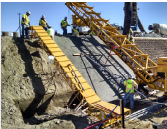
LEVEE CONSTRUCTION IN PUEBLO, COLORADO
