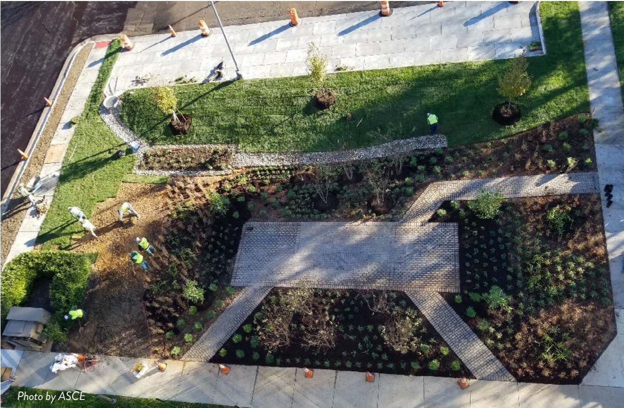
PERMEABLE PAVEMENT AND STORMWATER DETENTION IS BUILT INTO A PARKING LOT IN RESTON, VIRGINIA.
