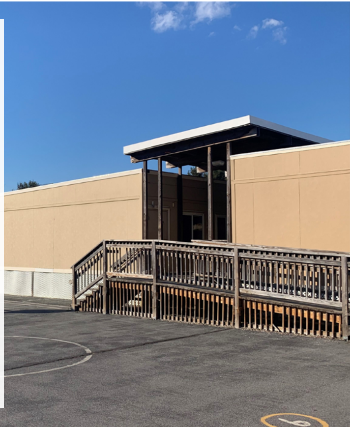
A TEMPORARY SCHOOL BUILDING IN MARYLAND.
