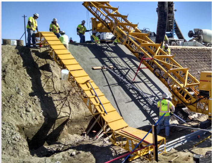
LEVEE CONSTRUCTION IN PUEBLO, COLORADO
