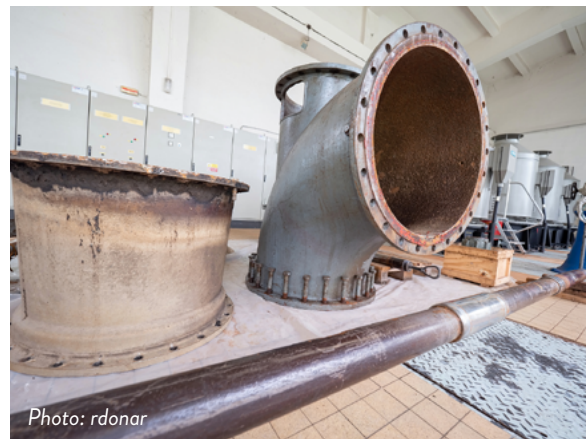
AXIAL HYDRODYNAMIC FLOW PUMP IN WASTEWATER PLANT.
