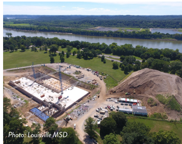
THE SOUTHWESTERN PARKWAY COMBINED SEWER OVERFLOW BASIN PROJECT
