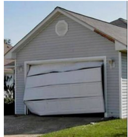
Garage door pulled out by the wind (click image for larger version)
