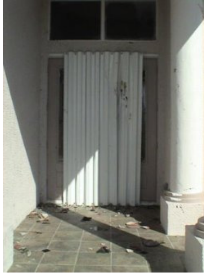
This shutter took a direct impact of a large tile missile. The door behind the shutter was damaged as a result.
