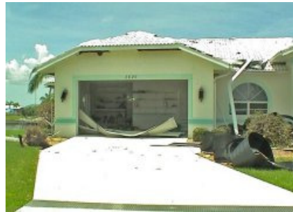
Garage door pushed in by the wind (click image for larger version)
