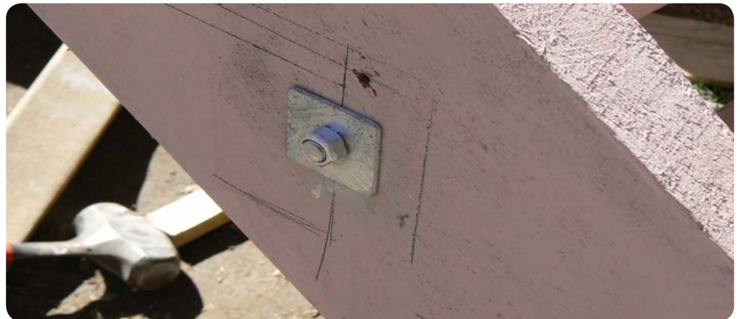
Figure 5.15: Position of step bolt.
