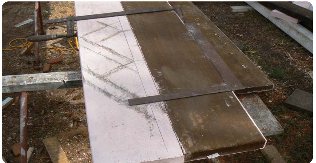
Figure 5.7: Marking out left string.
