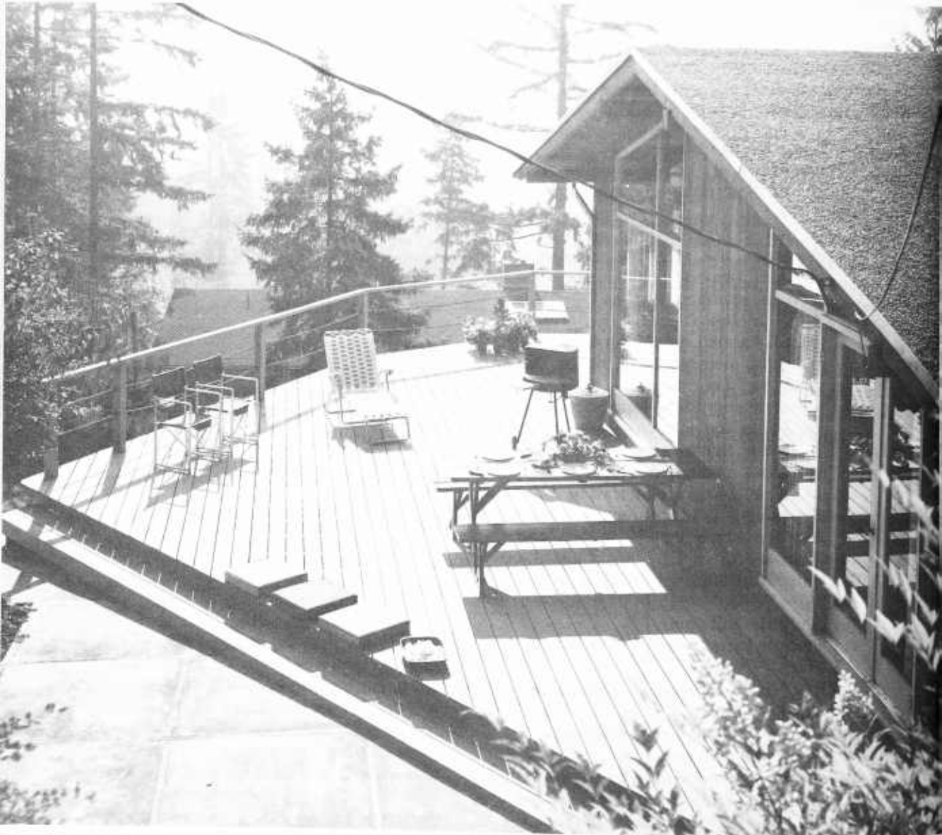
Figure 9. — Decks expand living areas on steep hillsides with little disturbance of the ground.
