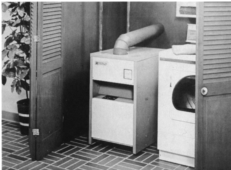
Figure 9-1 Electric-fired boiler. (Courtesy National Better Heating-Cooling Council)
