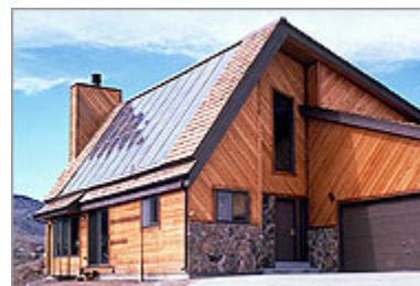
This home in Golden, Colorado uses a liquid-based solar system for space and water heating. Photo credit: Warren Gretz.
