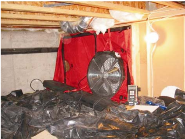
Fig. 5 Pressurization test in crawl space
