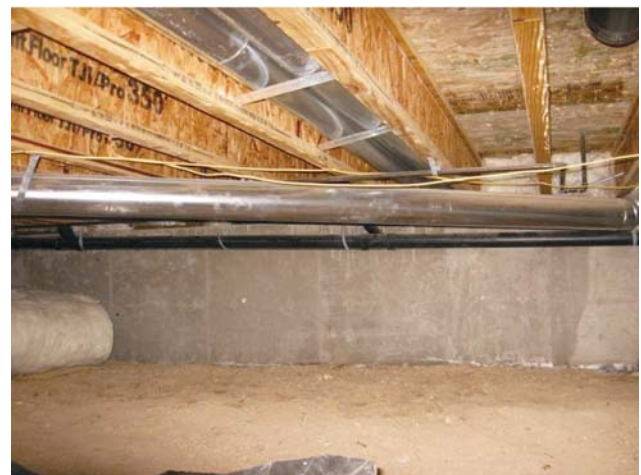
Fig. 2 Interior of crawl space A (no ground cover)
