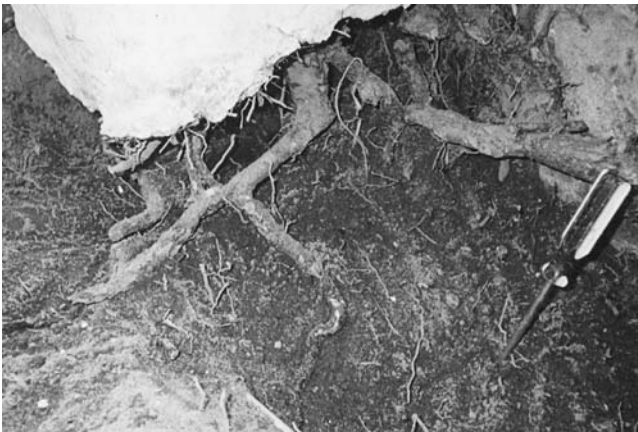
Fig. 14.4. Rhizomorphs of Meruliporia incrassata entering basement of home. Photograph courtesy of Luis De La Cruz (De La Cruz Wood Preservation Services, Van Nuys, CA).
