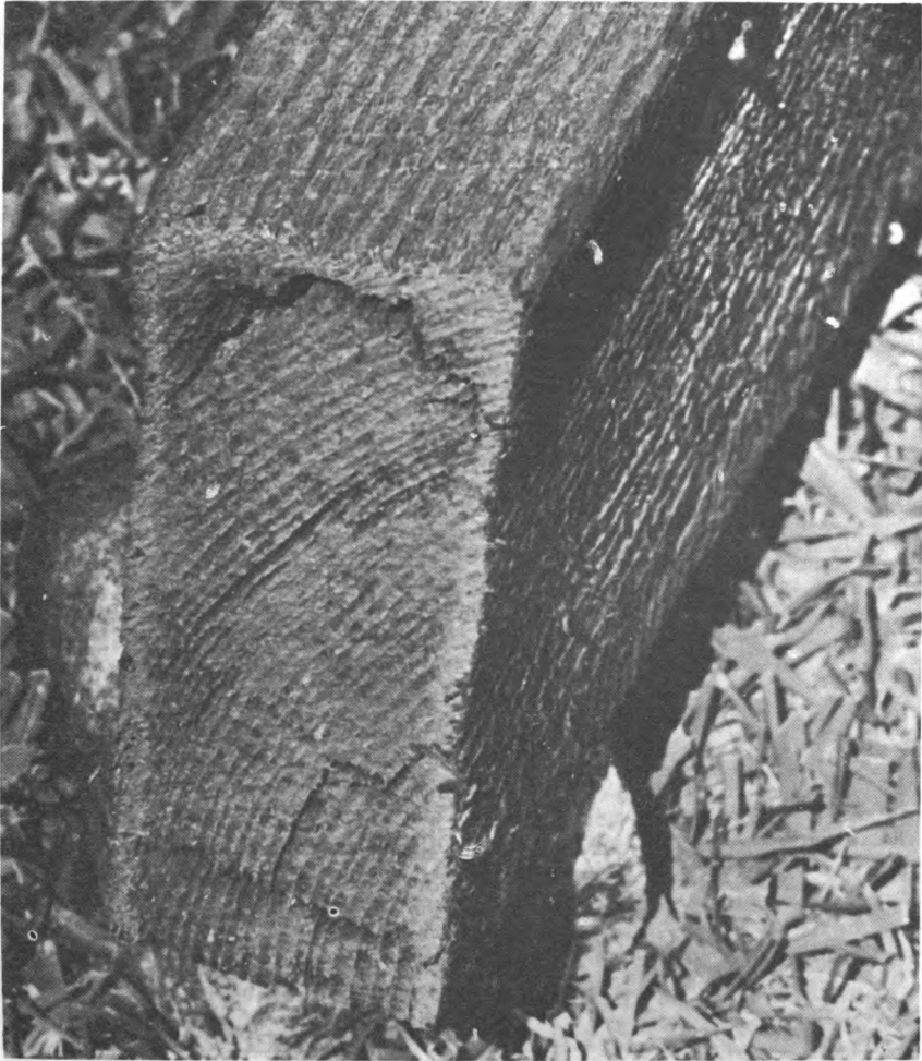
Figure 8. —Joist rotted by Poria incrassata in a dry crawl space; a sound shell of wood remains.
