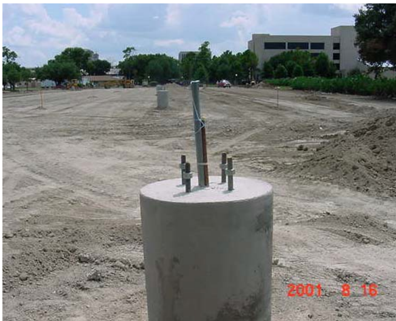
Figure 23 CONCRETE LIGHT POLE BASE WITH ANCHOR BOLTS
