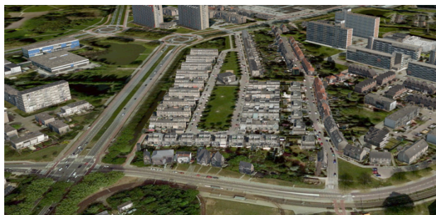
Figure 5 – 3D textured buildings in Rotterdam
