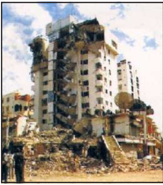
Fig. 3.3a: Destruction caused by an Earthquake in Gujarat
