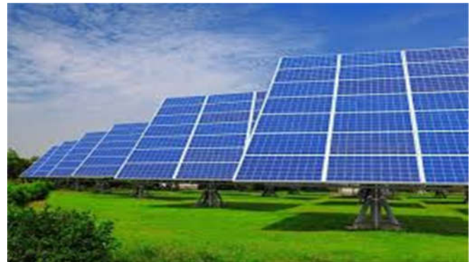
Figure 3. Solar power plant
