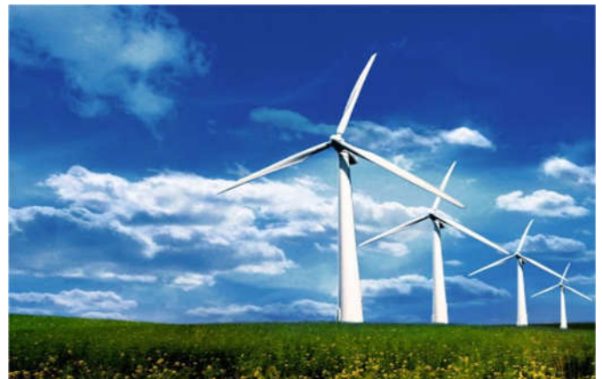
Figure 4. Wind power plant
