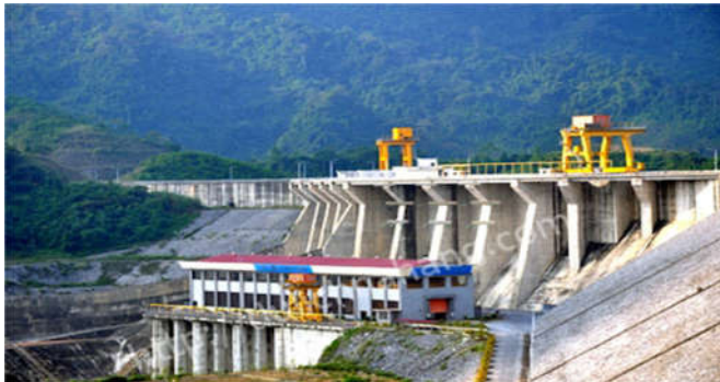
Figure 1. Hydroelectric power plant
