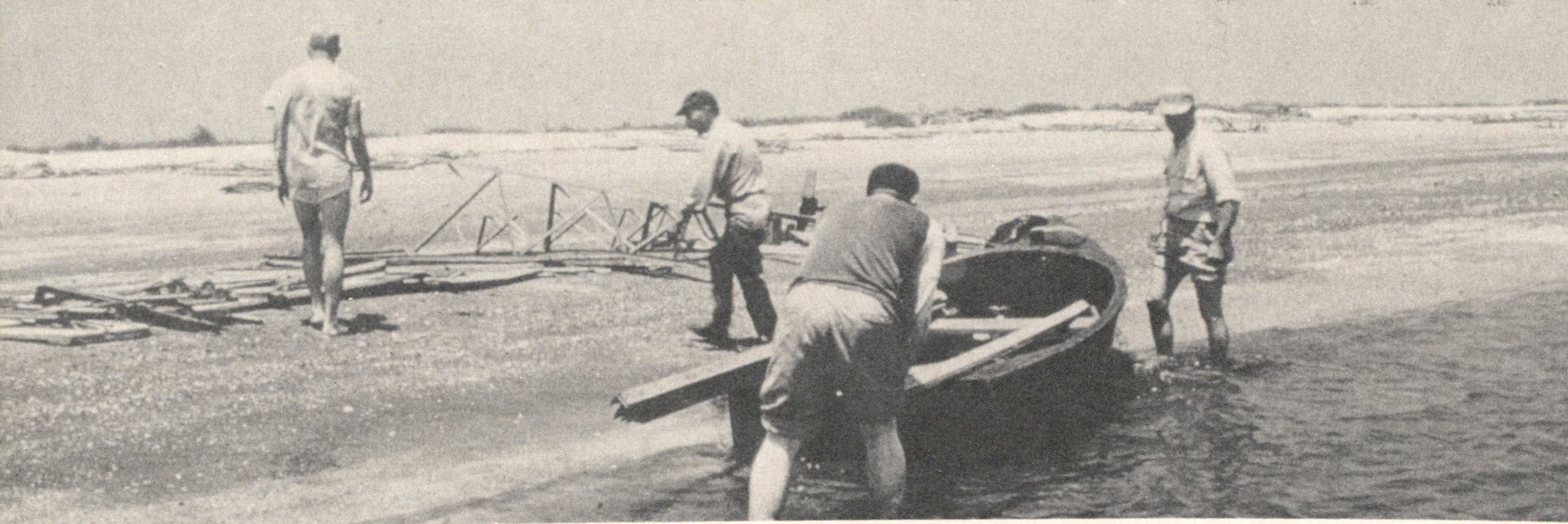
LIGHTERING STEEL TOWER MEMBERS ASHORE REQUIRED MANY TRIPS
