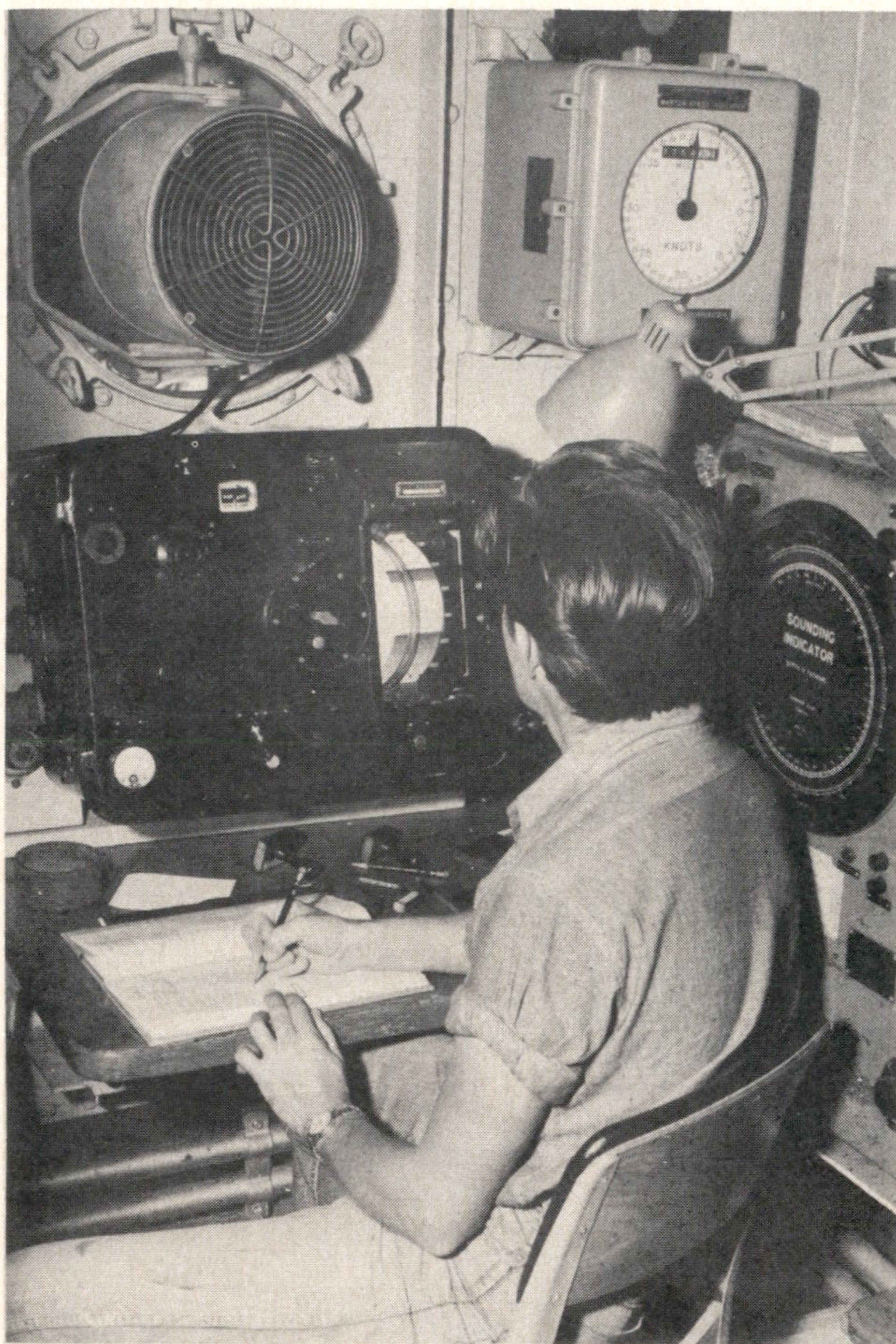
Type 808 portable graphic-recorder revolutionized sounding methods.
