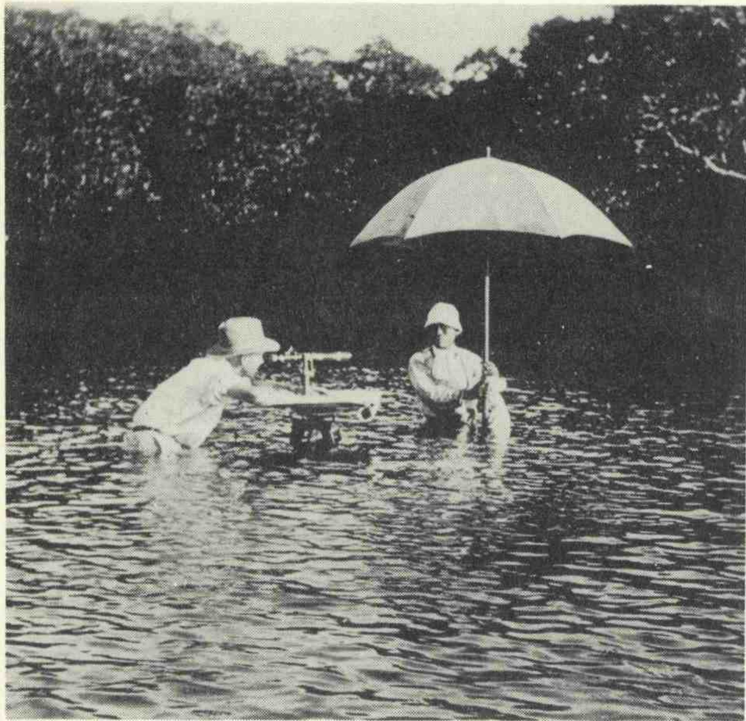
Planetable surveying in the Philippines
