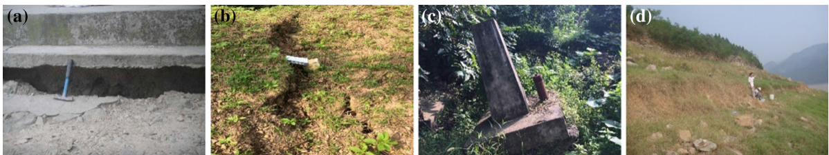
Fig. 5 Cracks in the landslide. a Crack C1, b crack C2, c crack C3, d crack C4
